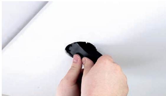
2 - quick connection box is placed over the 68 mm cut-out in the cavity
