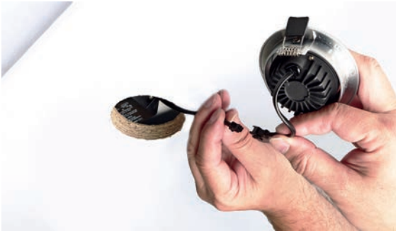
4 - connect the power supply unit to the spot using the connector
