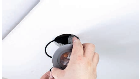
5 - inserting the spot into the ceiling cut-out
